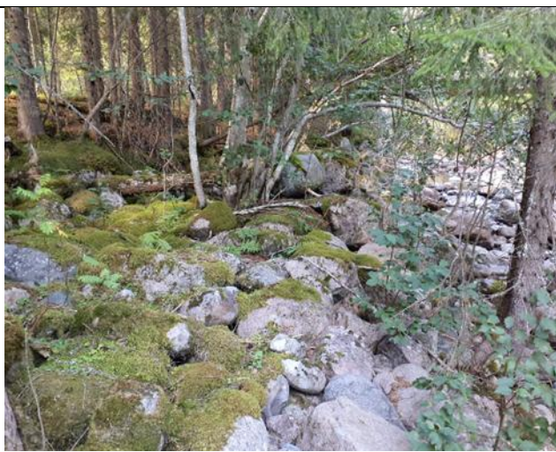
Figure 10. Example of vegetated boulder embankments that line much of the channel on both banks.
