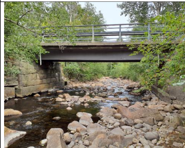
Figure 14. FV 120 road Bridge approximately mid-way along the study site. Looking downstream.
