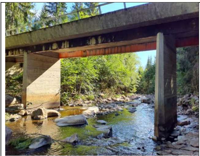
Figure 9. Bridge at the upstream extent of the survey area.
