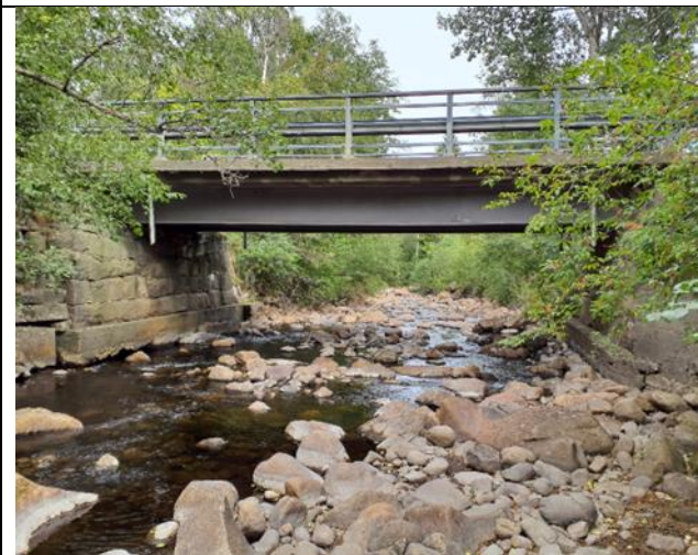
Figure 14. FV 120 road Bridge approximately mid-way along the study site. Looking downstream.
